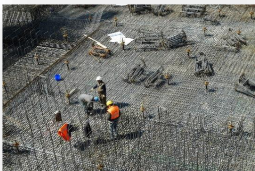
Electrical and Construction
